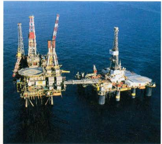
A Sedco Forex semi serving as a drilling tender in the Gannet field of the North Sea. Retrofitting of Sedco Forex rigs increases their ability to withstand years of service in rough weather, making them ideal candidates for the expanding market in tender-assisted drilling.
