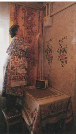
In Brovary, Ukraine, Galina Ivanova Pampuha, a Ukgas employee, reads a meter installed in her kitchen as part of a pilot project.
