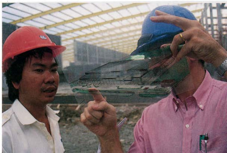
At the site of a new MEASUREMENT & SYSTEMS factory in Cikarang, Indonesia, Special Project Manager Bruno de Léotard, right, a mechanical engineer, with Sanjaya Atmaja, site manager for P.T. Indonakanogumi. De Léotard, a former Wireline engineer, coordinates construction of the multipurpose factory that will produce electricity meters, water meters, and pay phones for distribution in Asia.
